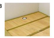
Remove the ply support and position the trap and connect to the wastepipe.
