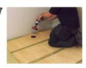
Using the pilot hole in the 18mm ply, cut a 100mm hole in the ply support for each trap.
