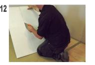
Trim the Graded Boards as necessary using a hand saw or similar.
