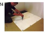
Fix the Graded Boards into position using the fixing washers provided.
