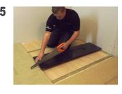
Where the grill is to be positioned against the wall, the Drainage Component is trimmed to 220mm along the premarked 'cut line'
