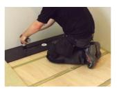
Screw the Drainage Component into place using the preformed screw holes.
