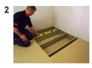
Check that all joists are level. Where necessary install noggins to support the edges of the wetfloor. Install timber battens 18mm from the top of the exposed joists.
